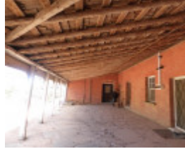
verandah of 1854 addition Sept 2015.JPG
