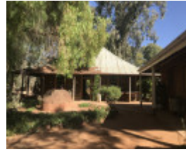
Rear Towannine Homestead
