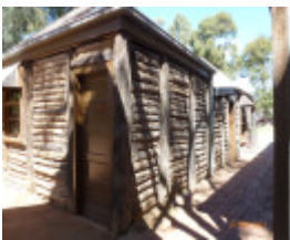
Rear of Post Office
