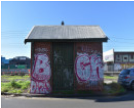
Colebrook Street substation
