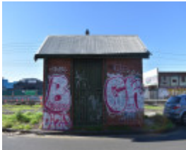
Colebrook Street substation
