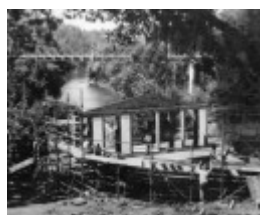
1983 Temporary scaffolded theatre for Epidavros Festival
