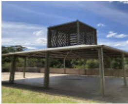
Gazebo Upper Level of Concrete Pavilion
