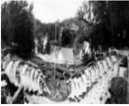
1985 Fairfield Amphitheatre during construction
