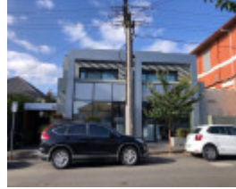
10-12 Llaneast Street, Armadale
