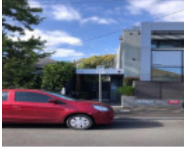
12 Llaneast Street, Armadale
