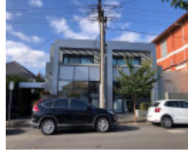
10-12 Llaneast Street, Armadale
