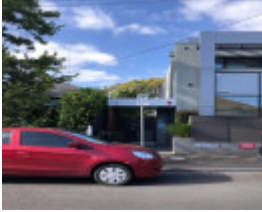
12 Llaneast Street, Armadale
