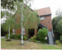
7 Mangan Street Balwyn
