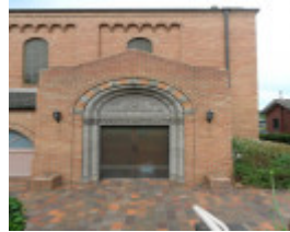
Former Frank Payton Memorial Church and Hall, 958A Burke Road Deepdene
