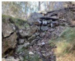
main trench overlooking road
