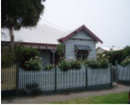
3 Storrer St, Geelong
