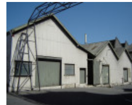
h01311 csr whitehall street yarraville engineers workshops 12 04 mz
