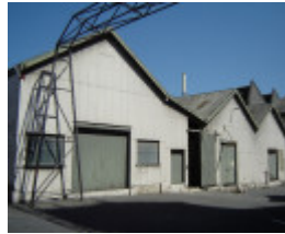
h01311 csr whitehall street yarraville engineers workshops 12 04 mz
