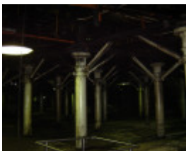
h01311 csr whitehall street yarraville interior south char end 01 12 04 mz
