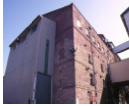
h01311 colonial sugar refinery whitehall street yarraville retail packing house
