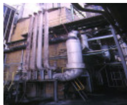
h01311 colonial sugar refinery whitehall street yarraville boiler house
