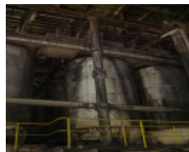
h01311 csr whitehall street yarraville interior south char end 02 12 04 mz
