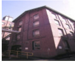
h01311 colonial sugar refinery whitehall street yarraville melting house
