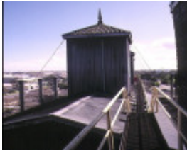
h01311 colonial sugar refinery whitehall street yarraville char tower
