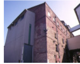
h01311 colonial sugar refinery whitehall street yarraville retail packing house
