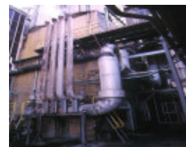
h01311 colonial sugar refinery whitehall street yarraville boiler house
