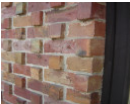
H2091 Lippincott House Glenard Dr Heidelberg Brick Detail Nov2005 mz
