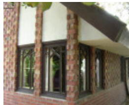
H2091 Lippincott House Glenard Dr Heidelberg Window Detail 04 Nov2005 mz
