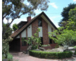
H2091 01 Lippincott House Glenard Dr Heidelberg Front Elevation 01 Nov2005 mz
