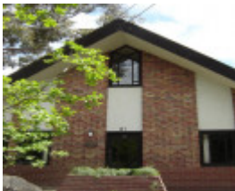
H2091 Lippincott House Glenard Dr Heidelberg Front Elevation 02 Nov2005 mz
