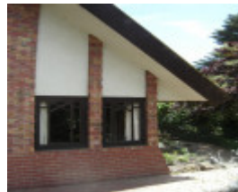
H2091 Lippincott House Glenard Dr Heidelberg Window Detail 02 Nov2005 mz
