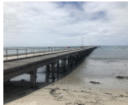
South side pier
