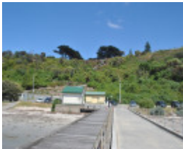
Cable landing site 2
