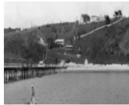
Pier staff quarters cable station 1890 1910
