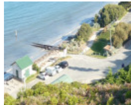
Pier boat ramp from above
