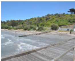
Cable landing site
