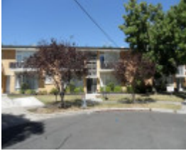
Ardene Court Flats, 11 Ardene Court, Hawthorn
