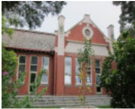
St Joseph's Catholic School (formerly St John's School), 571 Glenferrie Road Hawthorn
