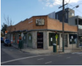
Belford Court Arcade, 54-58 Kilby Road Kew East
