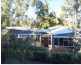
'Milston House', 6 Reeves Court KEW
