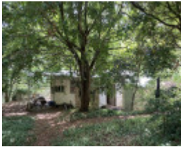
Edith Ingpen House View from Road Entrance
