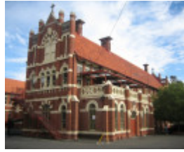
St Ignatius Church Richmond 3 May 2007 School North Wing
