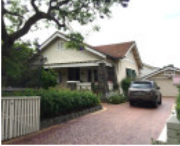
Adair House, 40 Havelock Road Hawthorn East
