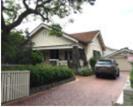
Adair House, 40 Havelock Road Hawthorn East
