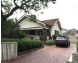
Adair House, 40 Havelock Road Hawthorn East
