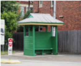
Tram Shelter (next to 441 Riversdale Road, Hawthorn East)
