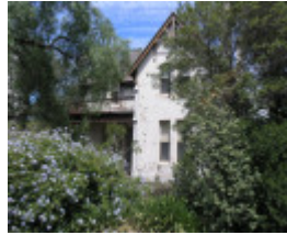
HOLY TRINITY CHURCH, VICARAGE AND HALL SOHE 2008
