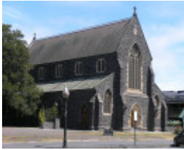
Holy Trinity Church, Vicarage and Hall SOHE 2008
