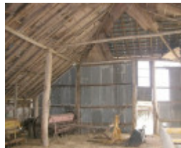
Staplegrove Meat Works Interior
