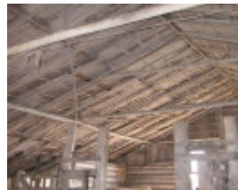
Staplegrove Meat Works Interior
