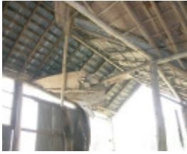
Staplegrove Meat Works Interior
