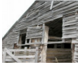
Staplegrove Meat Works Weatherboard Detail
