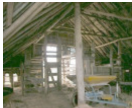
Staplegrove Meat Works Interior
