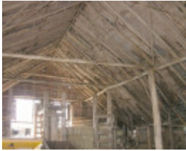
Staplegrove Meat Works Interior
