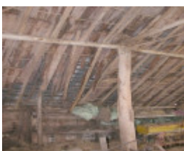
Staplegrove Meat Works Interior Framing
