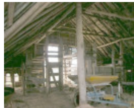
Staplegrove Meat Works Interior
