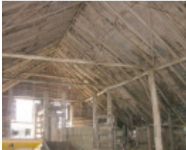
Staplegrove Meat Works Interior
