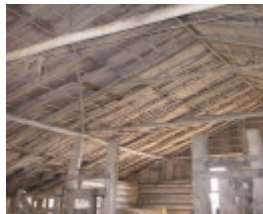
Staplegrove Meat Works Interior
