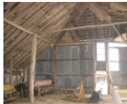
Staplegrove Meat Works Interior
