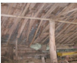
Staplegrove Meat Works Interior Framing
