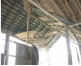
Staplegrove Meat Works Interior
