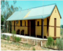
August 2022 Former Irymple Railway Station Building
