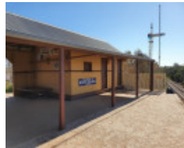
2020, Lobby and doors to the General and Ladies' waiting rooms
