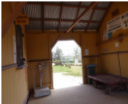
2022, Interior of lobby with ticket windows and remnant walls
