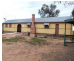
2022, Chimney side of building and edge of modern picnic shelter
