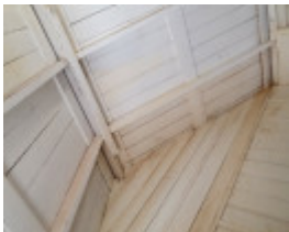
2020, interior of roof
