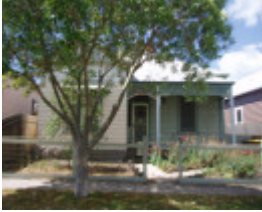
9 Thorne St, Geelong East
