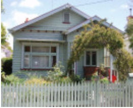
16 Thorne St, Geelong East
