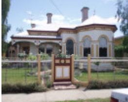
5 Verner St, Geelong South
