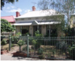
11 Verner St, Geelong South
