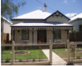
13 Verner St, Geelong South
