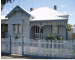
17 Verner St, Geelong South
