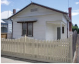
19 Verner St, Geelong South
