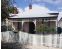
20 Verner St, Geelong South
