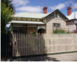
22 Verner St, Geelong South
