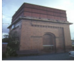
Elmore Railway Station Water Tower (1984)
