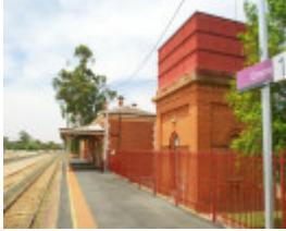
Elmore Railway Station and Water Tower
