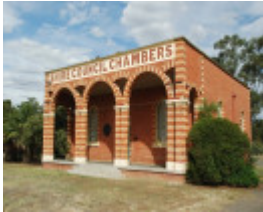
Former Huntly Shire Council Chambers
