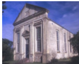
h00850 former st andrews presbyterian church and manse william st port fairy overall view she project 2003
