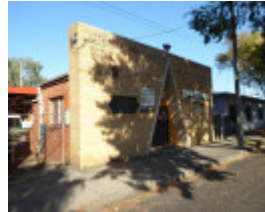
10th Caulfield Scout Hall August 2019-3-From East
