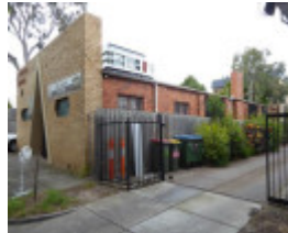
10th Caulfield Scout Hall August 2019-7-West Elevation
