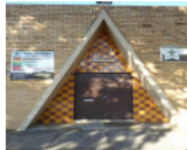
10th Caulfield Scout Hall August 2019-6-Front Entry
