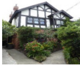
Duplex 21-23 Nepean Highway Elsternwick August 2019-4
