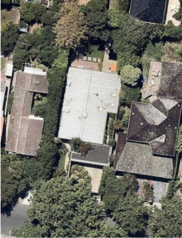
Edelstein Residence 13 Seymour Road Elsternwick August 2019-11-February2019
