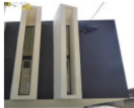
Elevated Townhouses 23 Seymour Road Elsternwick August 2019-6-South Facade
