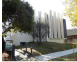
Elevated Townhouses 23 Seymour Road Elsternwick August 2019-3-South facade
