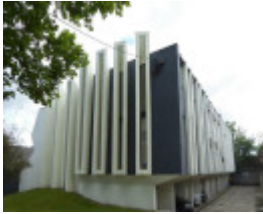
Elevated Townhouses 23 Seymour Road Elsternwick August 2019-1
