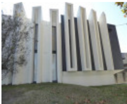
Elevated Townhouses 23 Seymour Road Elsternwick August 2019-5-South Facade
