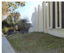
Elevated Townhouses 23 Seymour Road Elsternwick August 2019-7-South Facade
