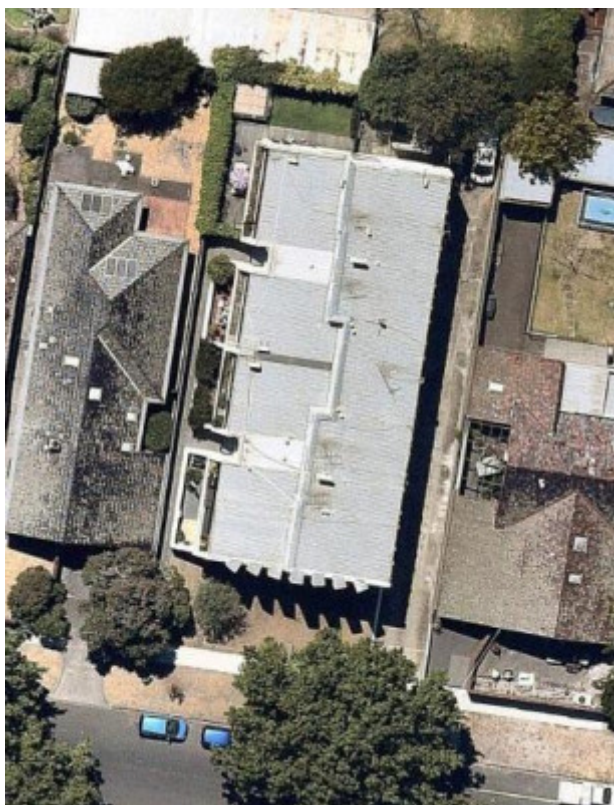
Elevated Townhouses 23 Seymour Road Elsternwick August 2019-15
