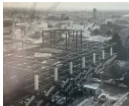
August 1977 the State Government Offices under construction
