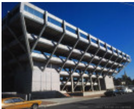
1979 State Government Offices viewed from Little Malop Street
