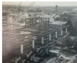
August 1977 the State Government Offices under construction
