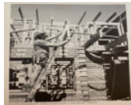
1982 - Kay Street Housing under construction - Housing Commission Annual Report
