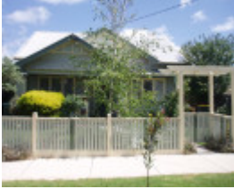
10 Winter St, Geelong East
