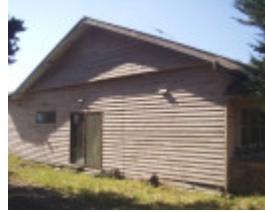
371-399 Lake Road, Connewarre - Exterior Side View
