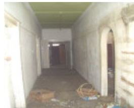
371-399 Lake Road, Connewarre - Interior Hallway
