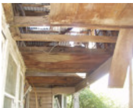
371-399 Lake Road, Connewarre - Exterior Verandah Roof
