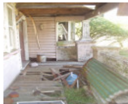
371-399 Lake Road, Connewarre - Exterior Verandah
