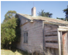
371-399 Lake Road, Connewarre - Exterior Side View - 2
