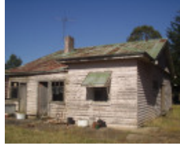
371-399 Lake Road, Connewarre - Exterior Back View
