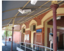
UPFIELD RAILWAY LINE PRECINCT SOHE 2008
