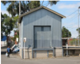
UPFIELD RAILWAY LINE PRECINCT SOHE 2008
