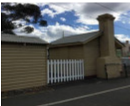
Park St gatekeepers cabin.jpg
