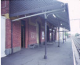
1 upfield railway line precinct parkville brunswick road brunswick platform
