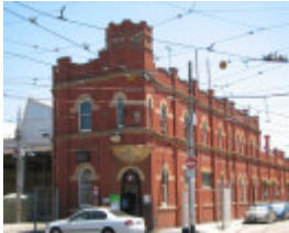
TRAM DEPOT SOHE 2008
