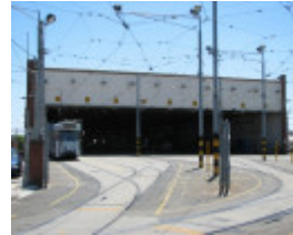
TRAM DEPOT SOHE 2008
