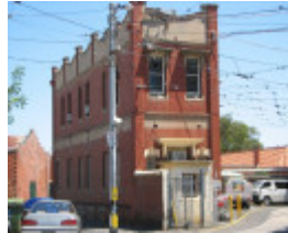
TRAM DEPOT SOHE 2008
