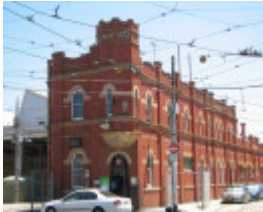
TRAM DEPOT SOHE 2008
