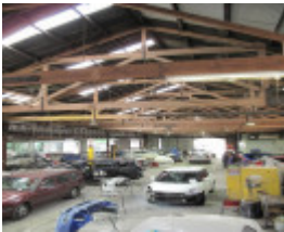
Northcote Tramways Building Thornbury May 2009 mz Engine House Interior 02
