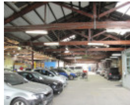
Northcote Tramways Building Thornbury May 2009 mz Car Shed Interior
