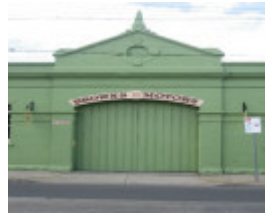
Northcote Tramways Building Thornbury Oct 2007 mz Car Shed Entry
