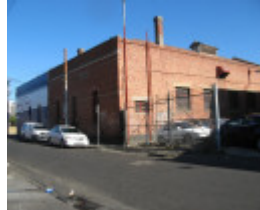
Brunswick cable tram engine house - substation
