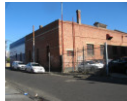
Brunswick cable tram engine house - substation
