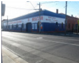
Brunswick cable tram engine house
