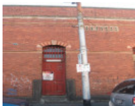
Brunswick cable tram engine house substation entrance
