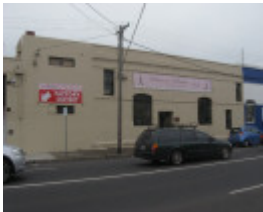
Brunswick cable tram engine house 261-63 Brunswick Road
