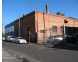
Brunswick cable tram engine house - substation
