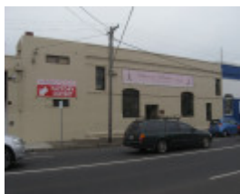
Brunswick cable tram engine house 261-63 Brunswick Road
