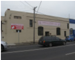
Brunswick cable tram engine house 261-63 Brunswick Road
