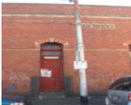
Brunswick cable tram engine house substation entrance
