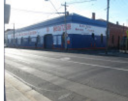
Brunswick cable tram engine house
