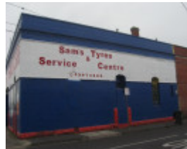
Brunswick cable tram engine house Black St facade
