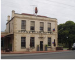
Fyansford Hotel - 67 Hyland Street, Fyansford - Exterior 1
