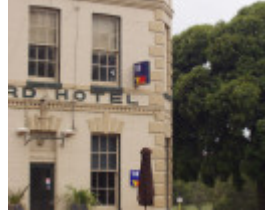
Fyansford Hotel - 67 Hyland Street, Fyansford - Exterior 2
