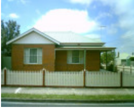
48 Ann Street, Geelong West
