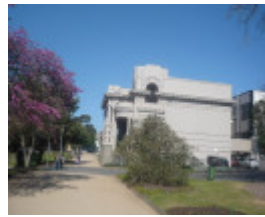
Johnstone Park Peace Memorial Building Side View
