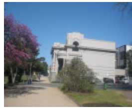
Johnstone Park Peace Memorial Building Side View
